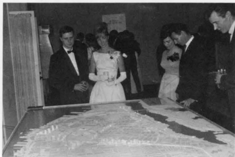
The New Halifax . . . Architects.
