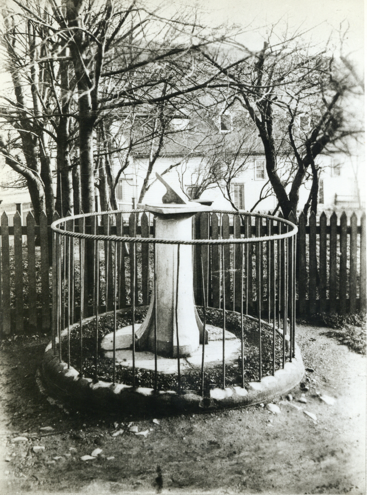
Sundial & Mast House H.M. Dockyard, Halifax (inside south gate)
