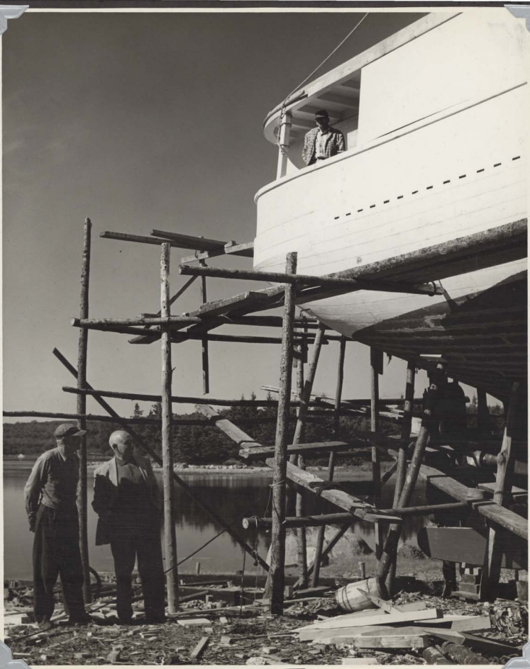
A NEW DRAGGER ALMOST COMPLETED.
