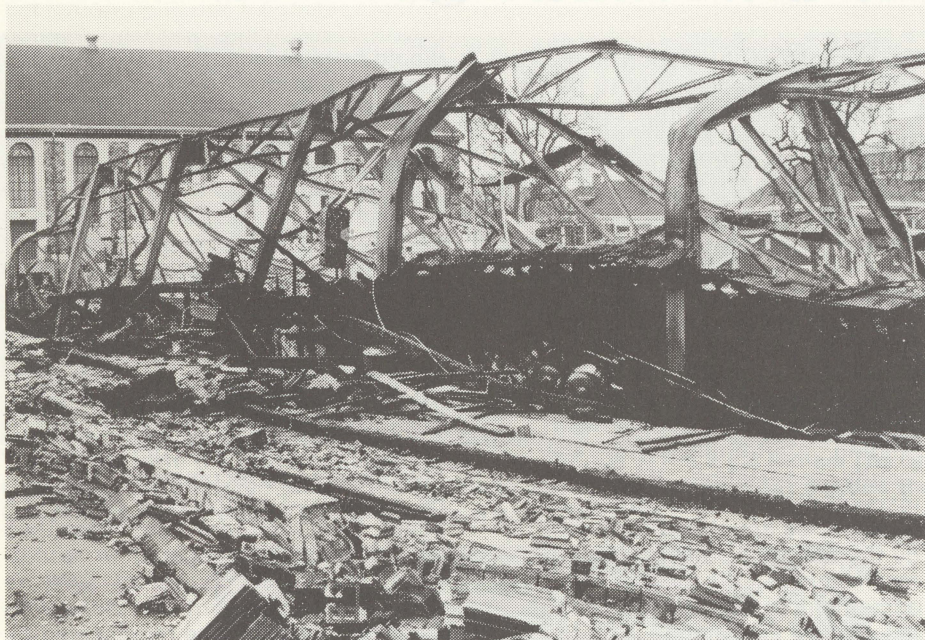
The twisted steel girders and rubble—all that remains.
