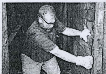
Tearing things up! Photo: EAC
