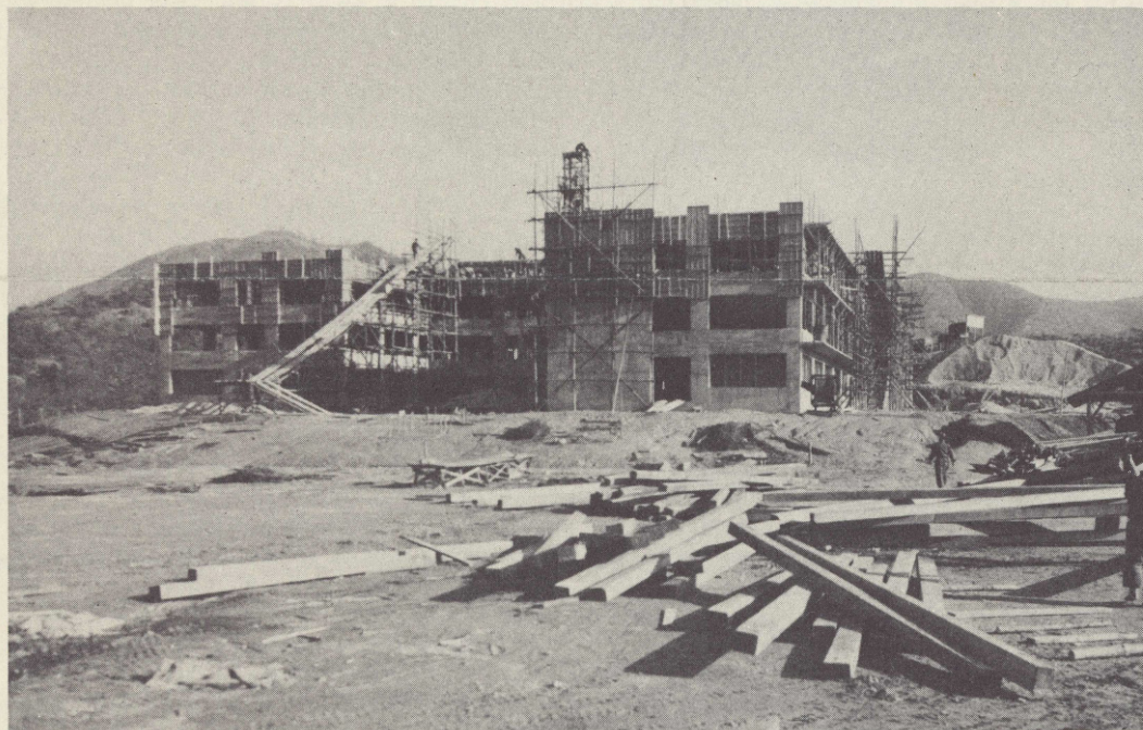
The Eighth U.S. Army Memorial Chest Hospital is already half built. The largest AFAK project will be completed by next summer. (U.S. Army Photo)
