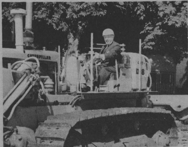
1965: Breaking ground for the Weldon Law Building.
