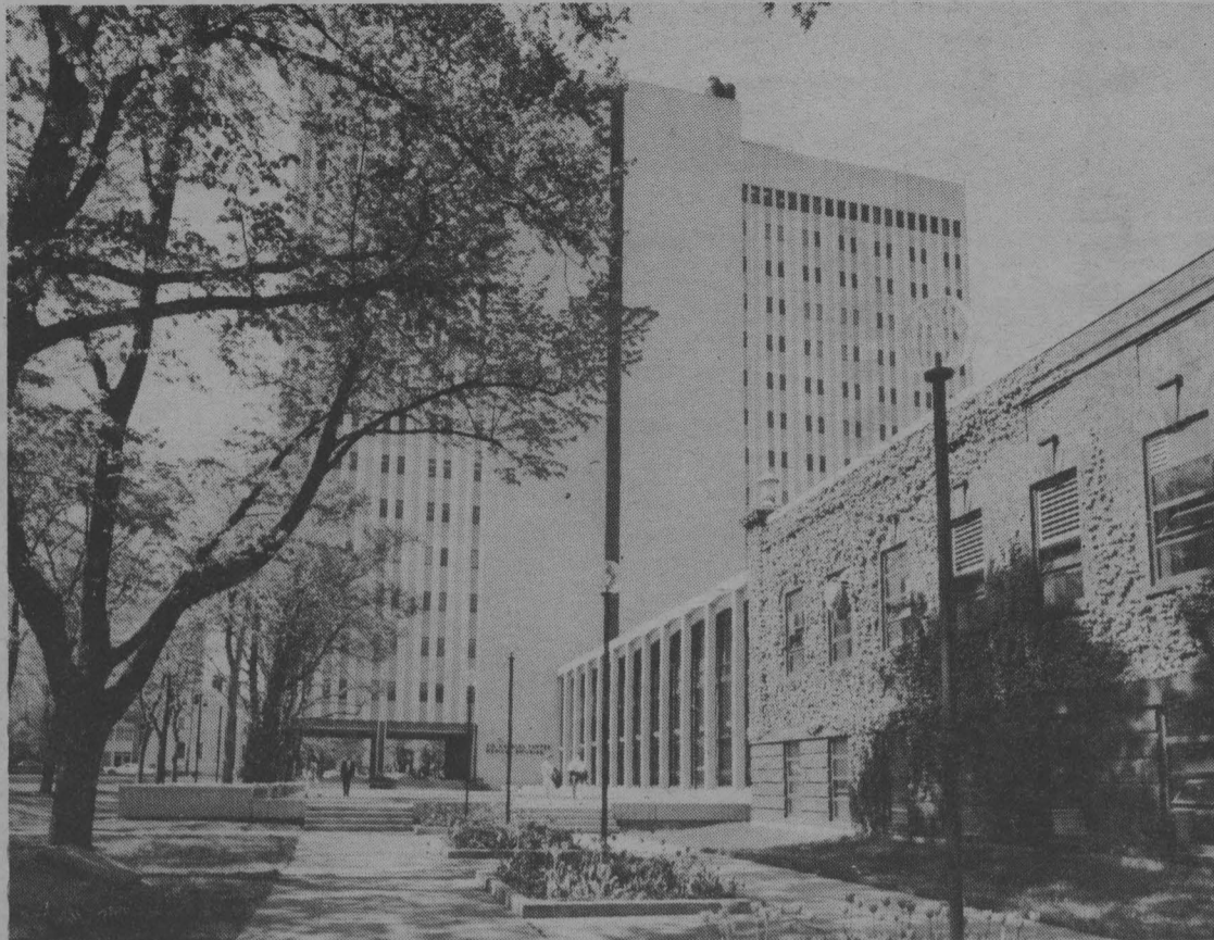
LEFT: The Sir Charles Tupper Medical Building, officially opened in 1967.
