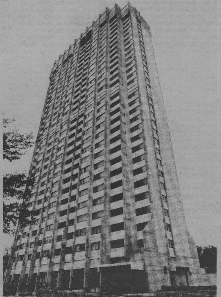
Fenwick Towers, an apartment building under construction, bought in 1971 as a student residence.
