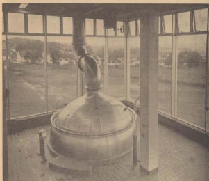
Large copper kettle with 7,500 gallon capacity.
