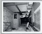
Preparatory work during the spring of 1983 included building a new electrical from for paper machine drive equipment, here shown near completion.
