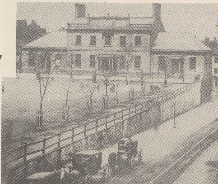
Dalhousie's first home on the Grand Parade site, where Halifax City Hall now stands. The carriages are on Barrington Street.
