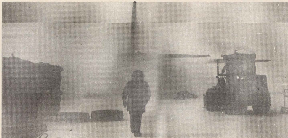
Snowmobiles and a bulldozer were dropped by parachute to the CESAR site and used to construct a runway on the ice for planes to land.
