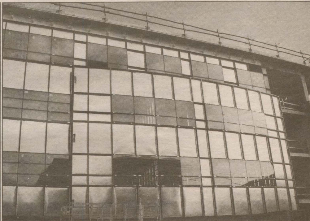
Studley campus' NA building, under construction | Photo by Andrew McCurdy
