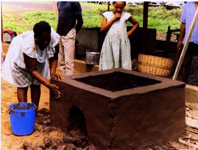
The "palayé" women of Neves formed a committee to manage their fish-smoking project. Here, the committee's president puts the finishing touches to a new Chorkor oven.
