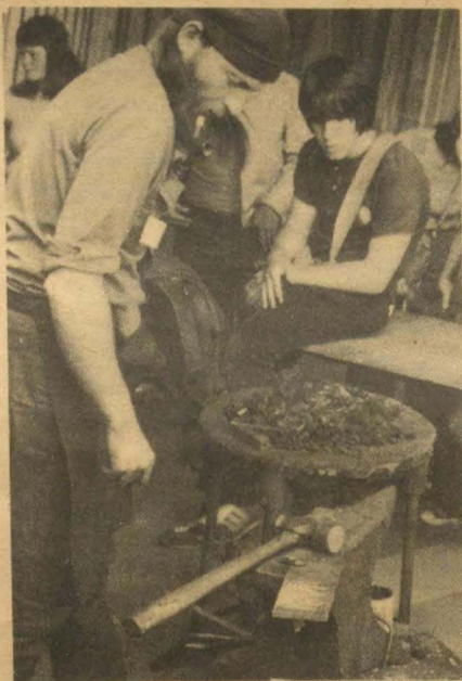
A Blacksmith at work
