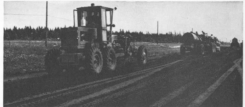
Soil Cement Highway, New Brunswick
