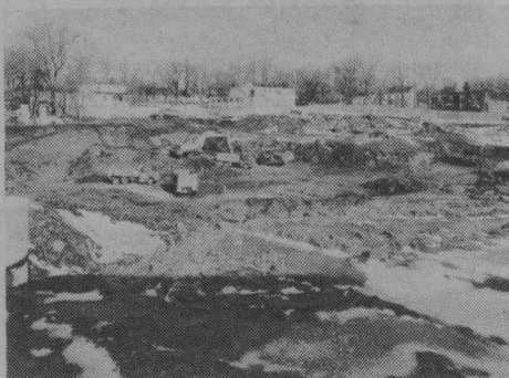
APRIL 1977: Digging the hole.
