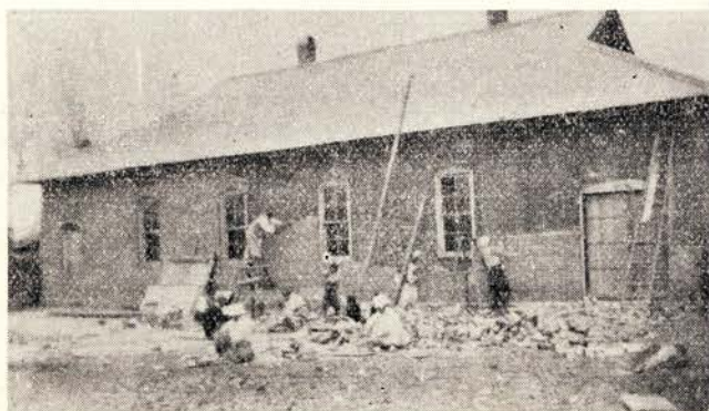
Removing the bricks from the old Central Church
