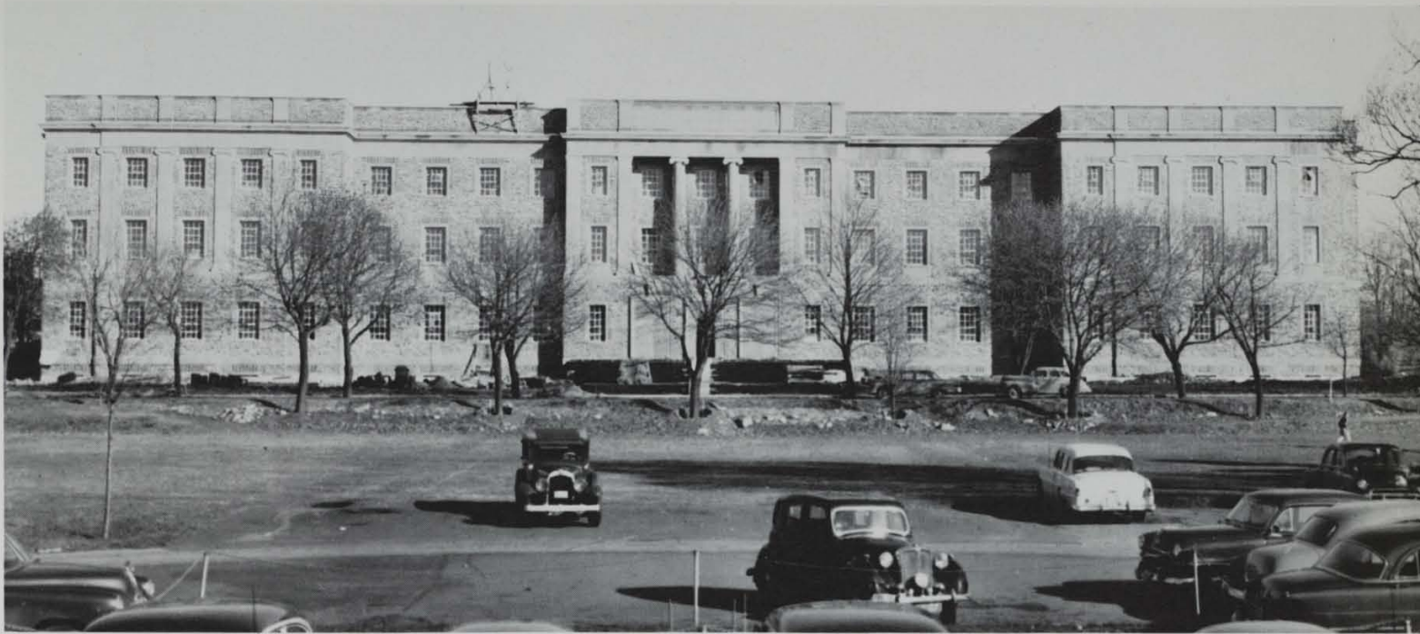
Shown above is construction on the Sir James Dunn Science Building in the early 1960's. It was a gift of the Sir James Dunn Foundation.
