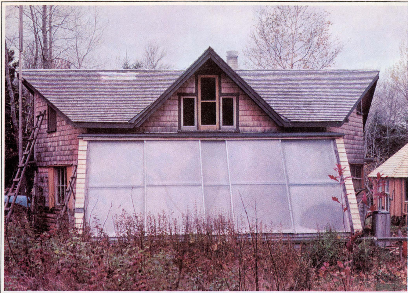
A steel-framed attached solar greenhouse enables Doug Miller and Denise Reiser of P.E.I. to pick fresh salads all winter.
