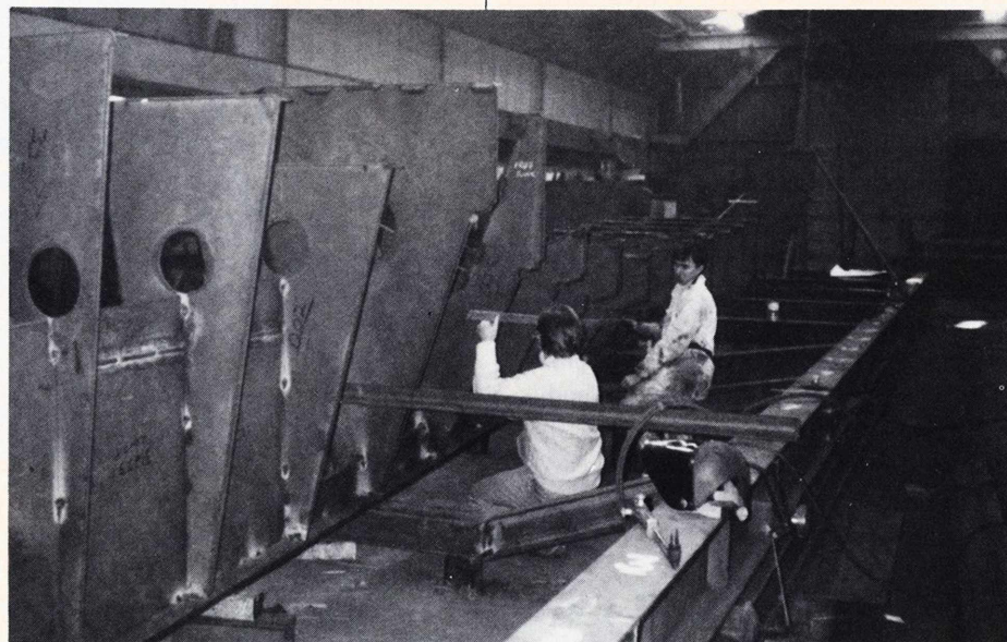
Floors installation on 65' steel wet fish dragger
