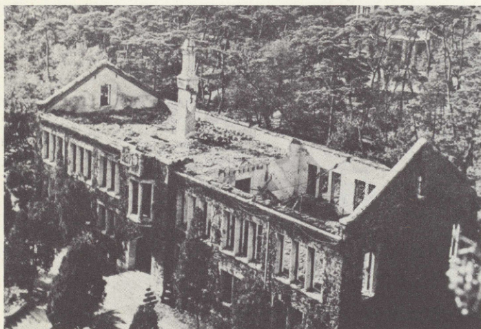
Shell and subsequent fire damage to Stimson Hall
