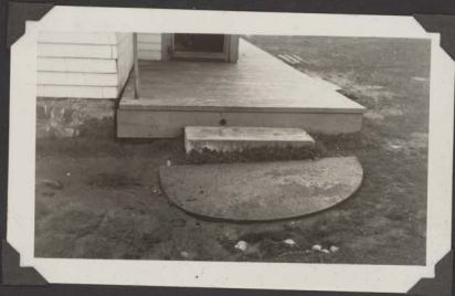
Lightkeeper's doorstep, Seal Island. Halfmoon iron plate is one of two made for original lantern base, to catch drip of seal oil used by Richard and Mary Richens in 1827.
