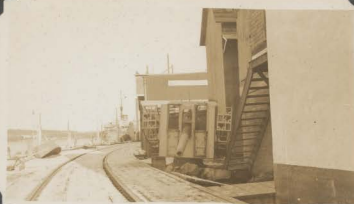
Liverpool waterfront, November 1945. 838 Note abandoned 4-inch gun, from a corvette.
